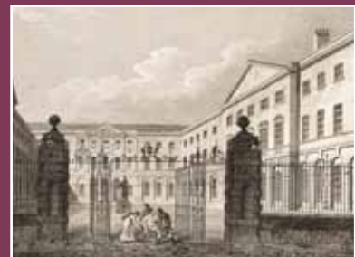
Guy's and St. Thomas' Hospital 1820.
